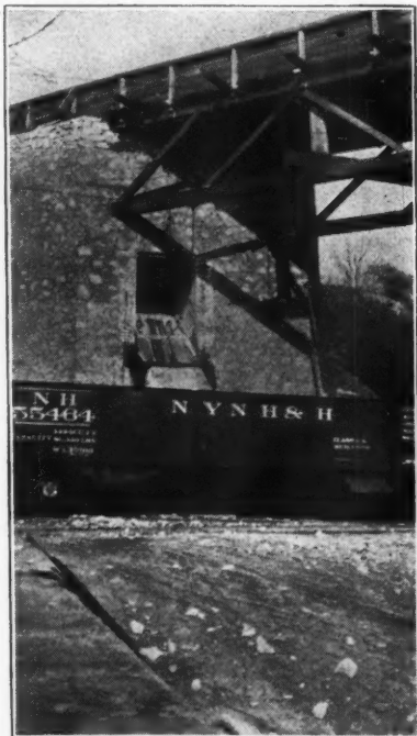
Chute for Loading Stone Into Cars.
